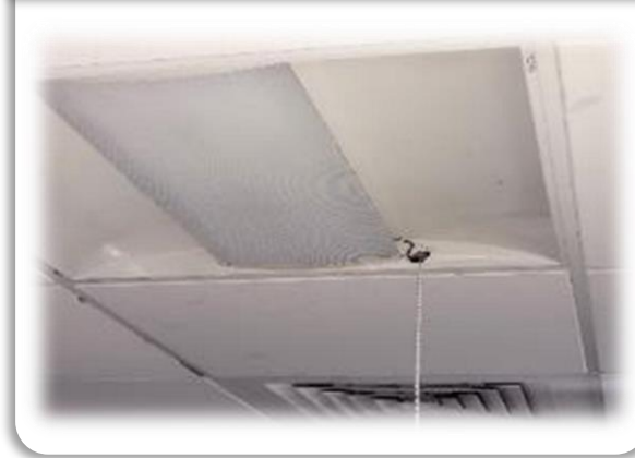
Pull Cord Switch Installation for Lighting
